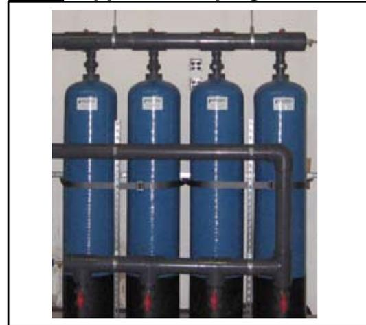
The full weight of the piping and valves must be supported by unistrut, pipe hangers or other means. The tank connections can not support the weight of the piping. This photo from a multi-tank system installation shows properly supported piping.
